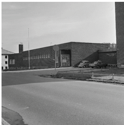
Elevator i Ole Deviks vei 20-22
